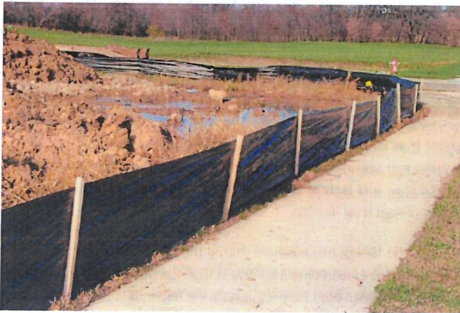
Figure 6.2 Typical Silt Fence to be Employed
